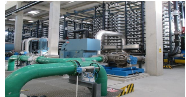
Use of non-conventional resources: desalination plants
