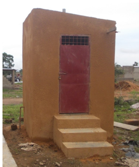
Latrines Ecosan © Association Koassanga
