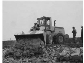
Lead wire gabion loading and casting by excavator
