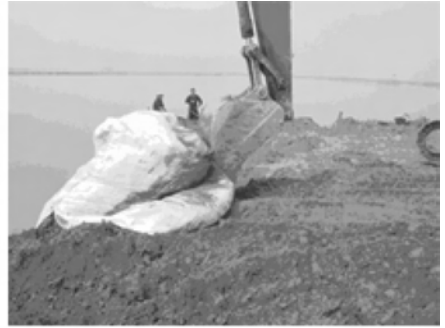
Fig. 1 Geocontainer pushed by a bulldozer Fig. 2 Geocontainer pushed by an excavator
