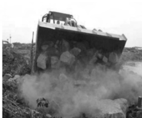
Stone unloading on the fascine
