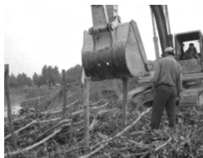
Piling by excavator
