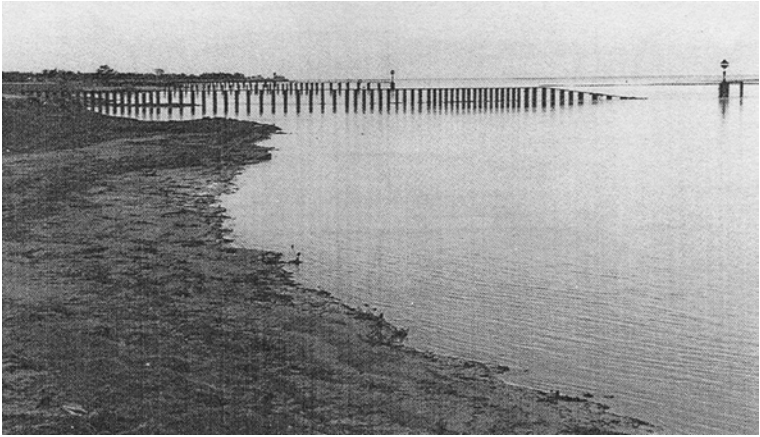
Fig. 4 Pile row in a pilot project along the Brahmaputra River in Bangladesh, 1996 (Wal, 2001)
