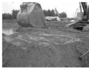
Levels off by excavator
