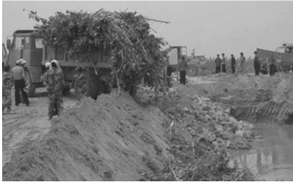
Wicker and stones pillow encroaching by dump truck
