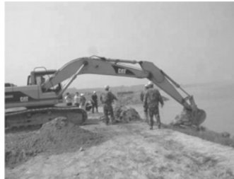
Lead wire gabion loading and casting by loader
