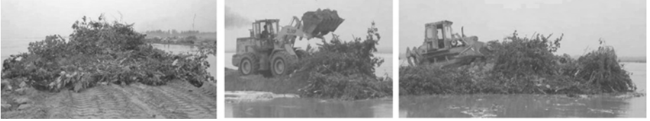
Spreading the soft material by forklift loading stones by loader Blend with wicker and stone
