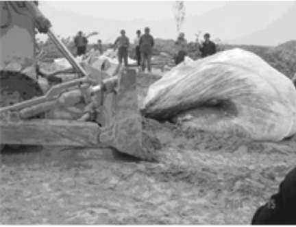
Fig. 1 Geocontainer pushed by a bulldozer Fig. 2 Geocontainer pushed by an excavator
