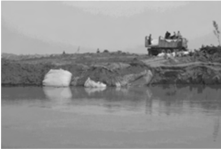
Fig. 7 Underwater execution of large geotextile
