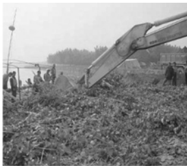
Fascine surface handling by excavator
