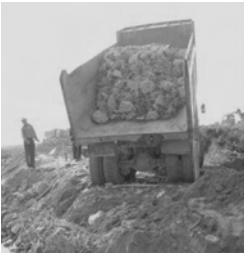
Lead wire gabion casting by dump truck
