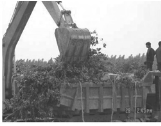
Loading soft material using excavator
