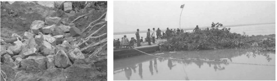
Put stones behind the fascine
