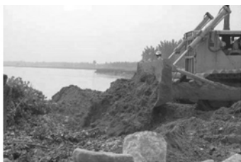
Fascine encroaching by bulldozer
