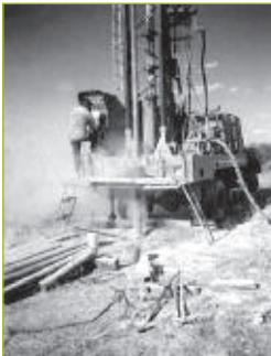
Drilling a well
